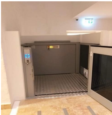
Figure 9: platform lift found inside the First-floor galleries.
