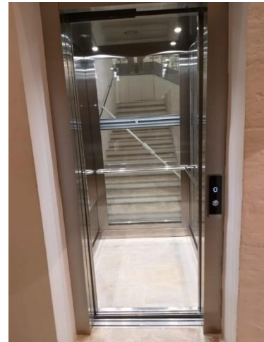
Figure 8: lift next to the staircase (found at Ground floor level).
