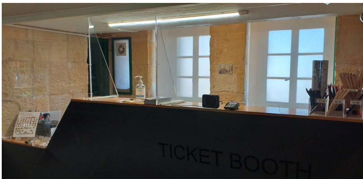
Reception desk with two heights for more accessibility. Also equipped with Perspex for health and hygiene and also microphone and speaker system.
