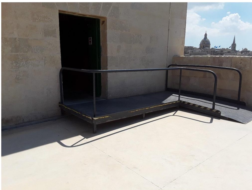
Ramps with handrails where entrances or exits are not at a floor level
