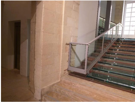
Figure 6: Staircase + the lift on the left side of the picture (found at ground floor level).
