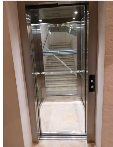
Figure 7: lift next to the staircase (found at Ground floor level).
