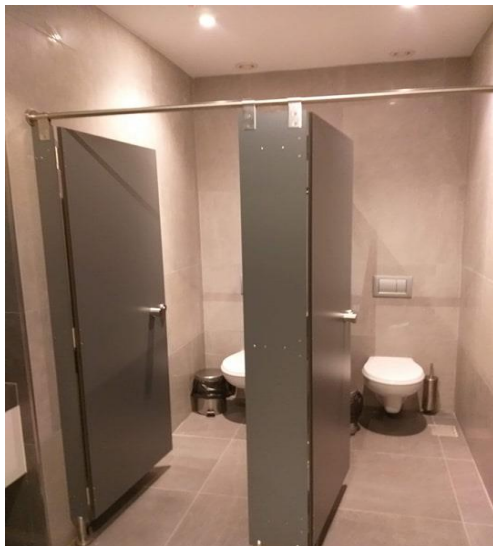
Figure 12: First Floor Ladies Restroom
