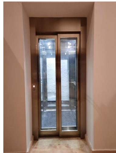
Figure 9: Elevator found in first floor galleries
